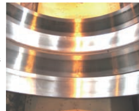
Hardly any indication of rust
