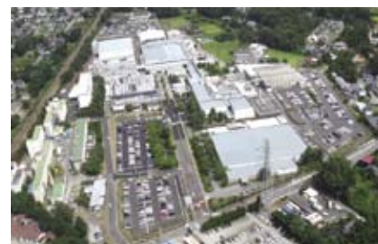
Fujisawa Plant / Japan
